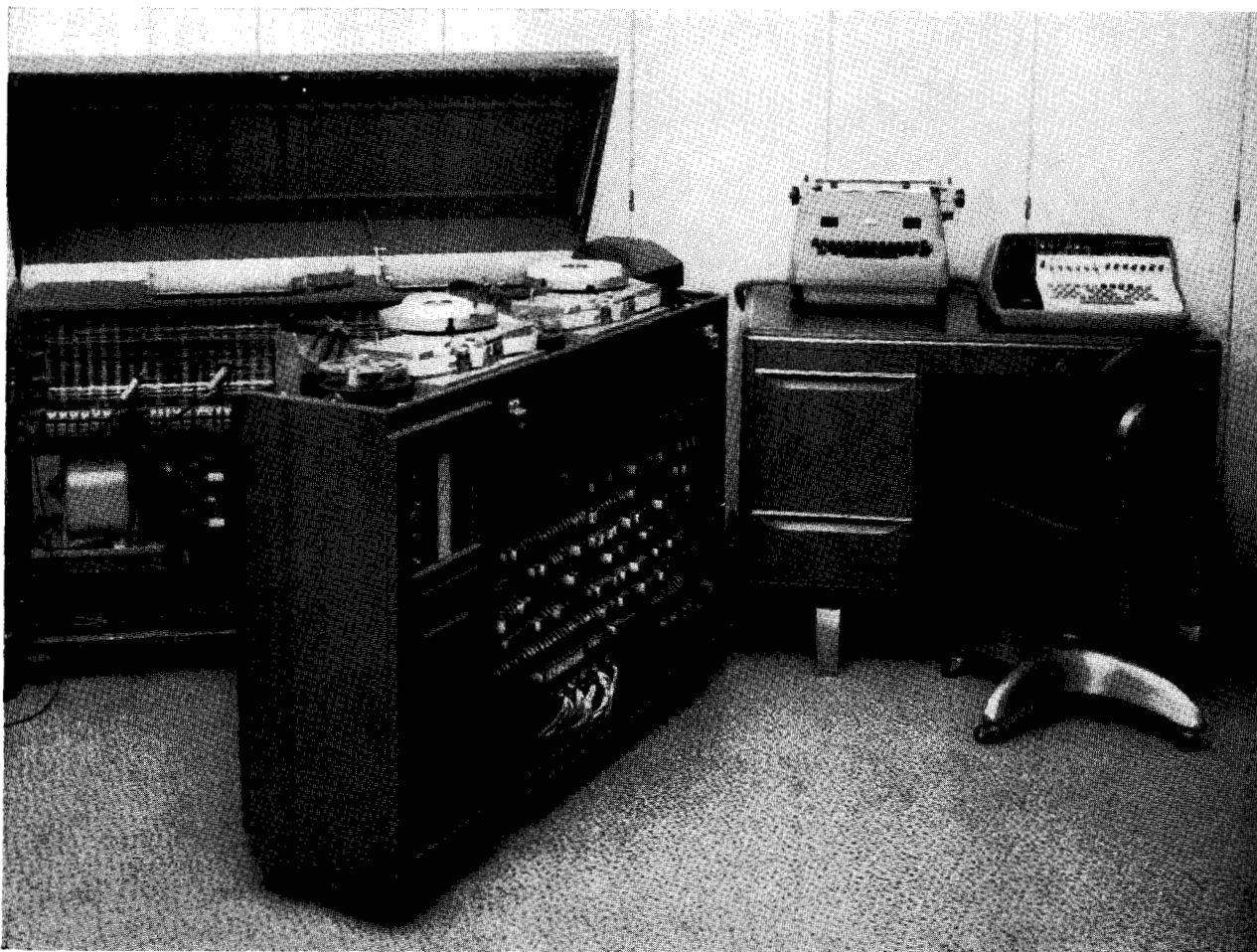
Figure 1 The computer opened to show construction.
