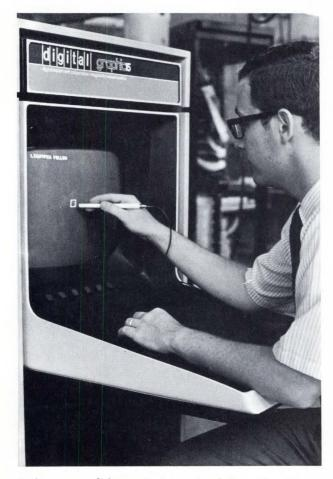
**Engineer uses a light pen for interactive design** with a softcopy display device. For this application, a refresh display is required. The system, Graphic 15, is built around the PDP-15 computer.
