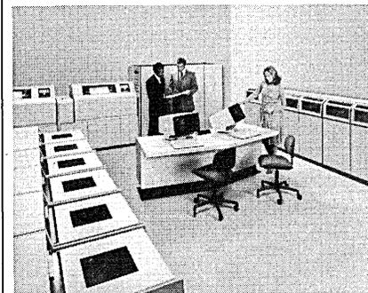
Both members of the family have cycle times of 28nsec. The V-8650 has a 32KB cache, and 96KB of instruction storage unit memory; the dual processor V-8670 has 128KB of cache, and 192KB of instruction memory. The instruction storage unit, loadable from diskette, can optimize the system for FORTRAN or COBOL environments. The V-8650 can have 4MB
