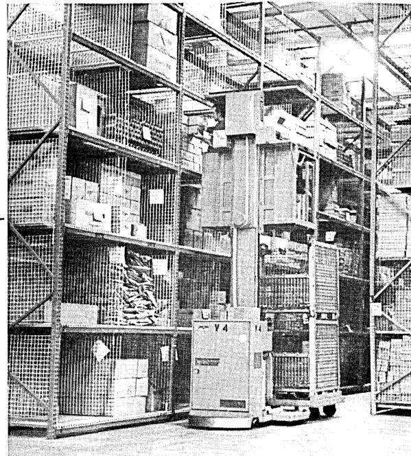
Mobility Systems' guided order-pick vehicles installed at Ford Motor Co.'s North American parts redistribution center automatically carry order pickers to the correct location. Vehicles can be directed by manual keyboard data entry, on-board punched card readers, or on-line computer.
