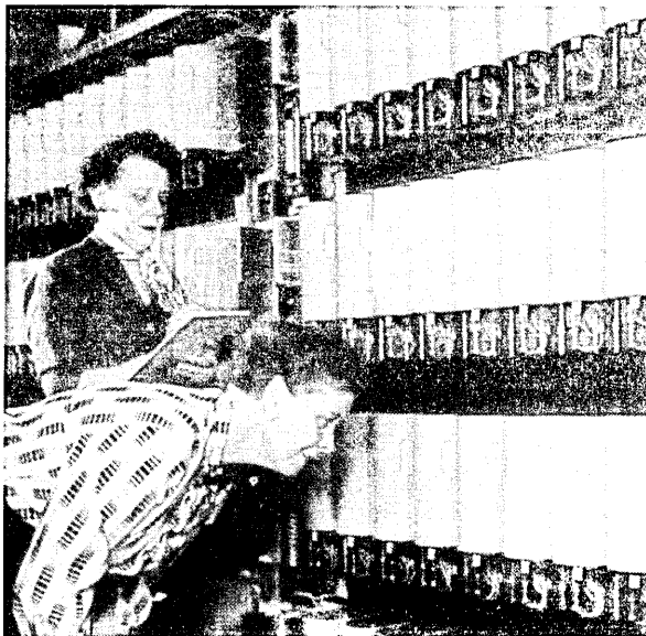
Fig. 1—A manual count being recorded of number of switches engaged with calls. The count was made to determine usage in SXS dial offices.
